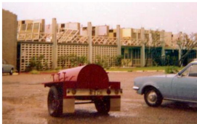
The old WRANS Quarters at HMAS Coonawarra immediately after the cyclone showing how the roof had been blown off and the walls of the upper floor had collapsed.
